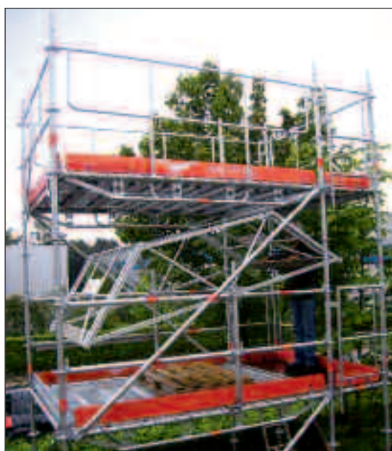
guardrail fits into 2.0 m, 2.5 m or 3.0 m deep loading bays
